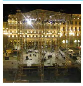
The lifter uses QL76A trusses. It was designed to withstand the stresses that large structures transfer to the ground in their heaviest duty use.
