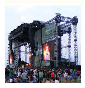
LITEC has deigned the MyT LED screen ground support to fly very heavy screens. The load bearing capacity is 12,000 kg on a maximum height of 20 m.
