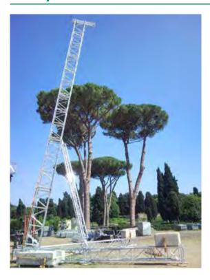
Support Tower for audio systems consisting of a QX40SA structure, suitable for lifting loads of up to 750 kg to a height of 7.5 metres or a QH40SA structure, suitable for lifting loads of up to 900 kg to a height of 9.5 metres. To lift the loads, anchoring is provided for an electric chain hoist.
