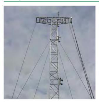
Vertical audio system support tower. It consists of QL52A structures and is suitable for lifting loads of up to 2500 kg to a height of 13 metres.
